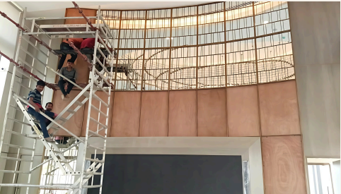
Feature wall installation in progress on site
