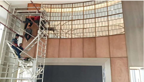
Feature wall installation in progress on site
