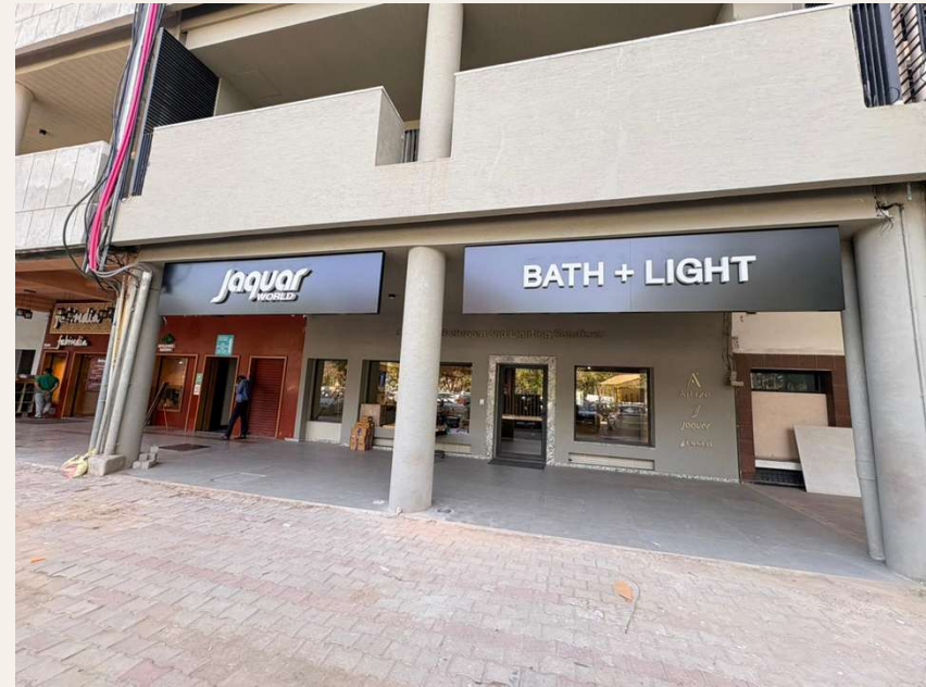
Bath + Light building front
